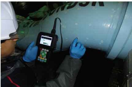
Carbon steel piping wall thinning inspection
