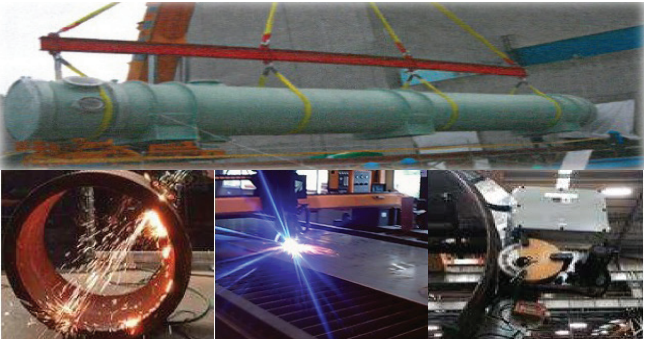
Decommissioning and decontamination of nuclear facility
