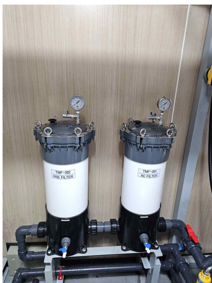
(e) Pre-filter and activated carbon fiber filter
